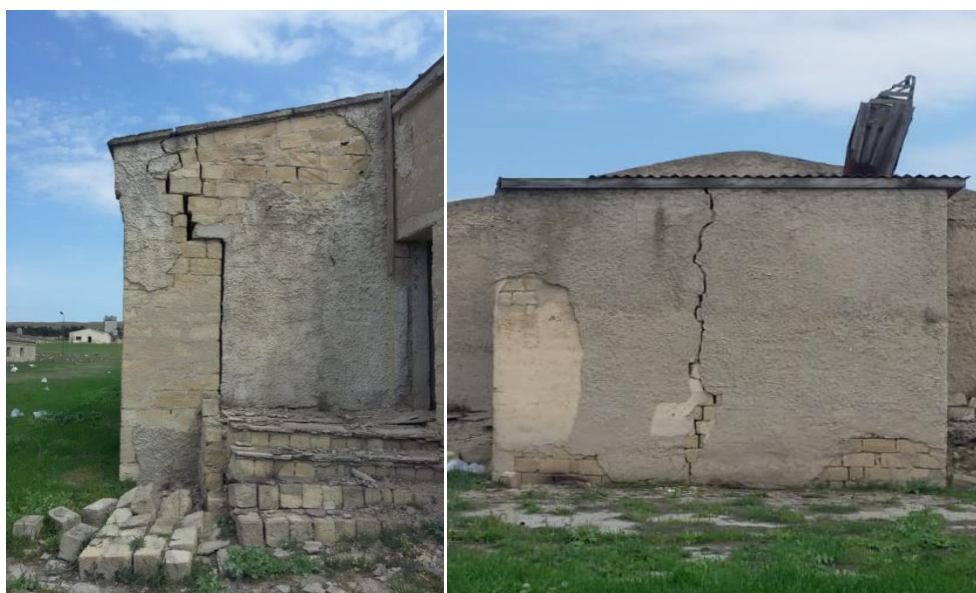
Figure 6. Damage caused by volcanic eruptions on a farm near the foot of the Gobu-Bozdagh volcano.
