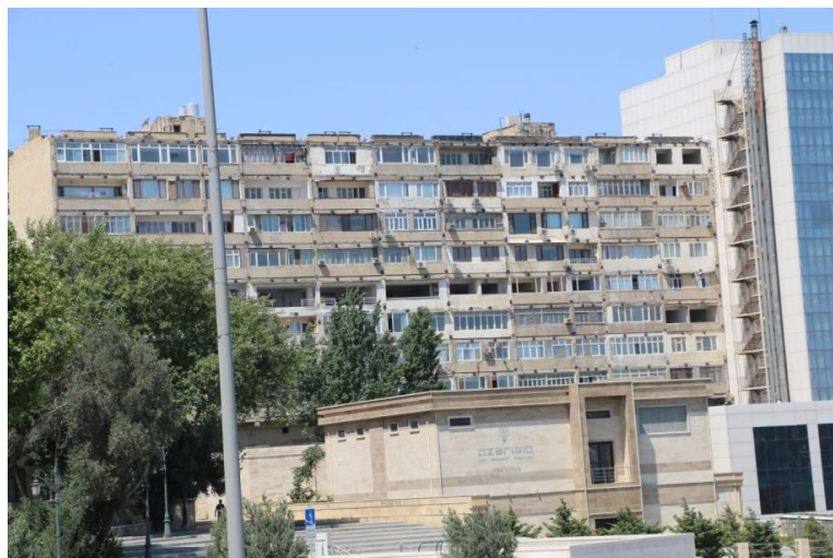
High-rise 9 storey buildings built in the past (during Soviet times)
