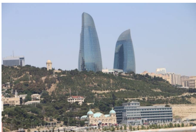
Bayil landslide area
