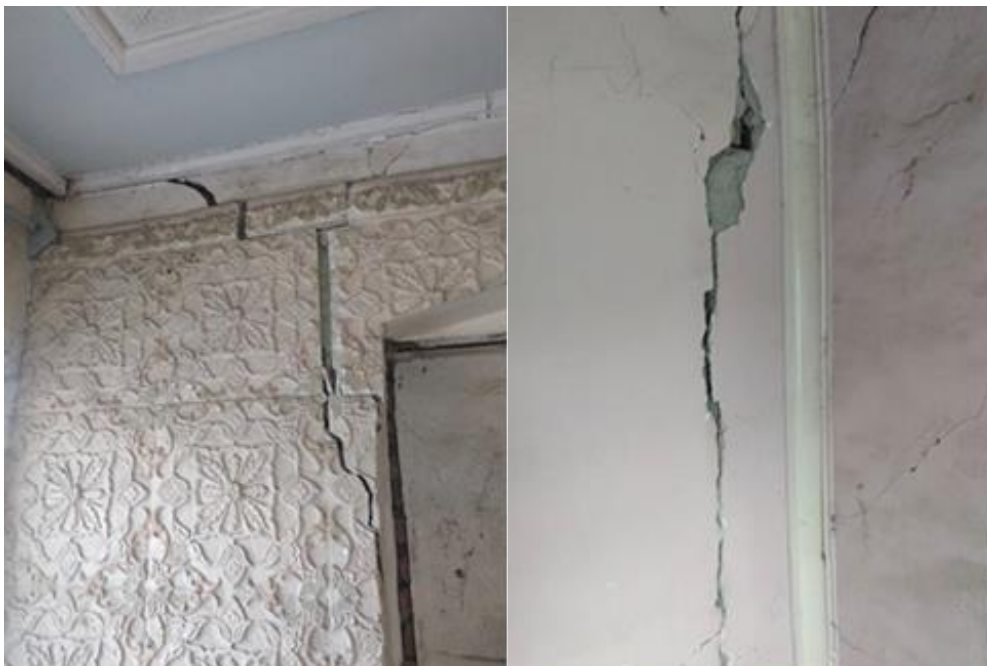
Figure 7. Old and new cracks on the wall of a house in Goyam village
