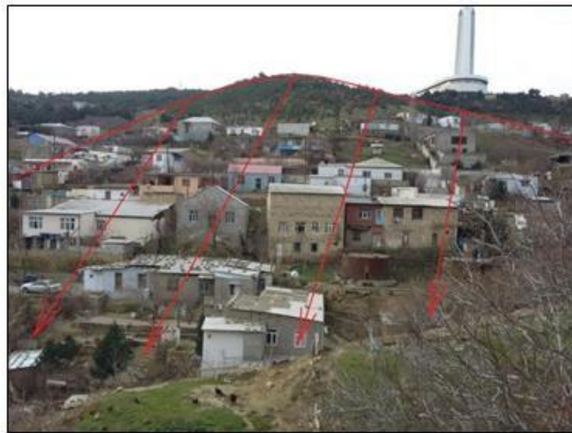
Fig. 2. View of houses in the affected area of the prognosed landslide (width 200 m, length 220 m).
