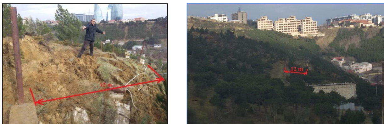
Fig. 16. Relocation of a stone fence
