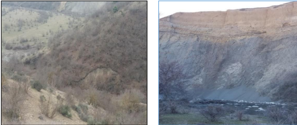
Figure 3. Local landslide and fall areas observed in the reservoir area. Engineering-seismic exploration works
